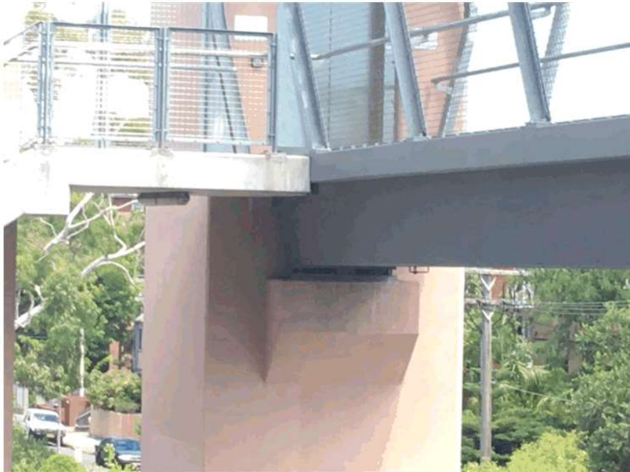
Bland Street Pedestrian Bridge – Southern abutment and bearing
