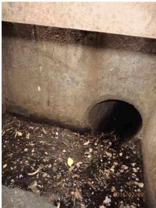
Stormwater drain pit and outlet downstream from DP-090
