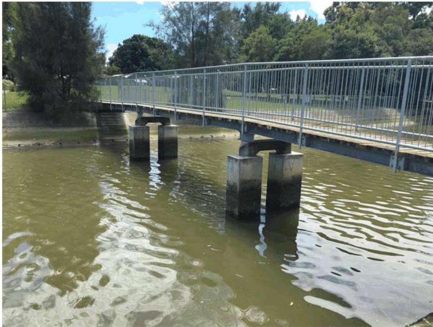
Wattle Street – Iron Cross Creek Pedestrian Bridge – Piers
