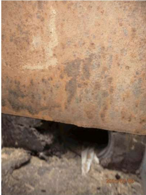
Drain outlet appears to be unblocked.
