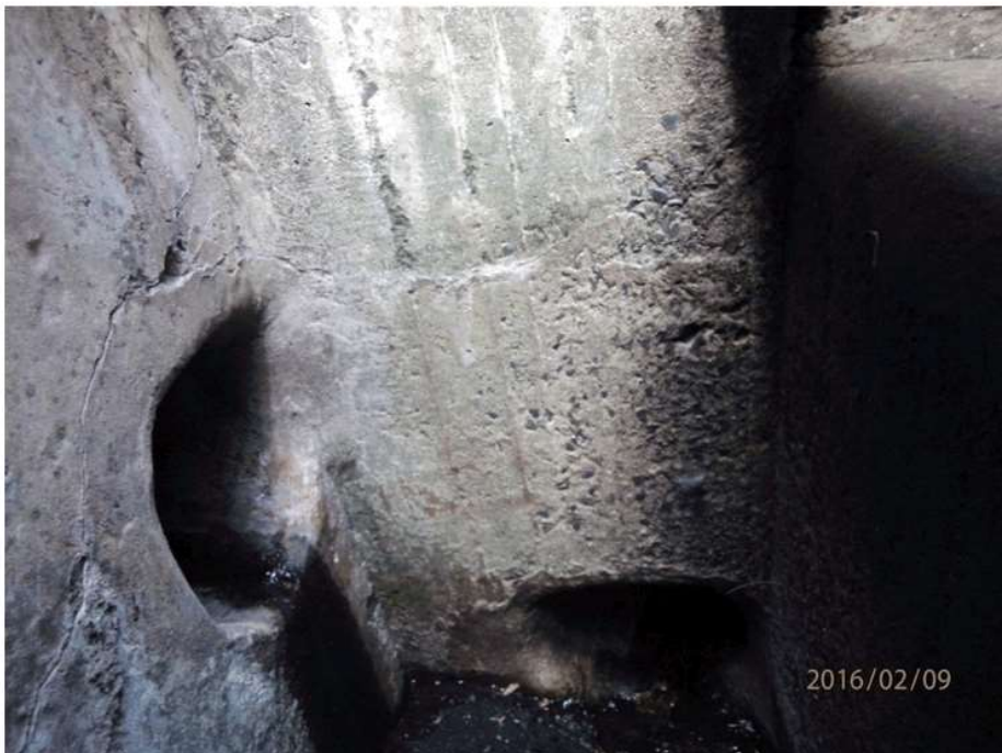
Drain inlet and outlet
