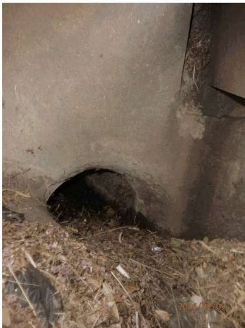
Stormwater drain pit and outlet
