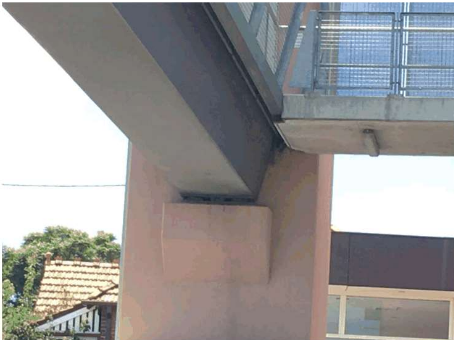
Bland Street Pedestrian Bridge – Northern abutment and bearing
