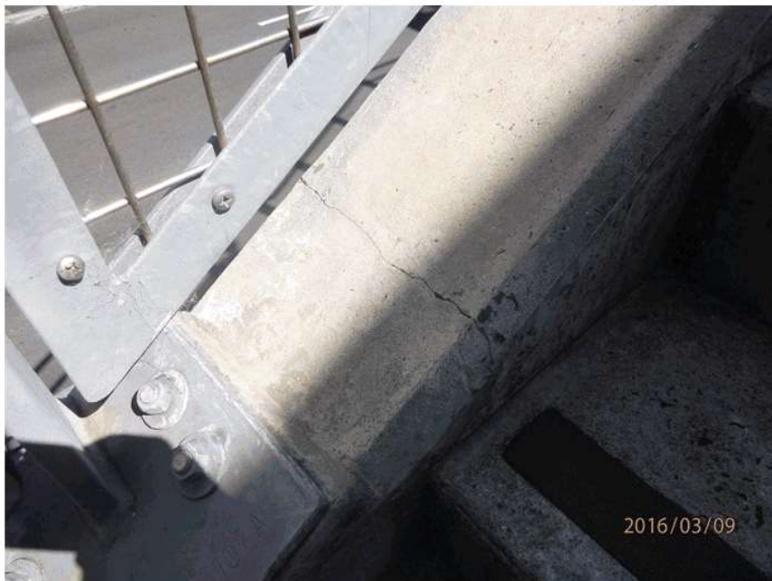
Bland Street Pedestrian Bridge – cracked northern staircase
