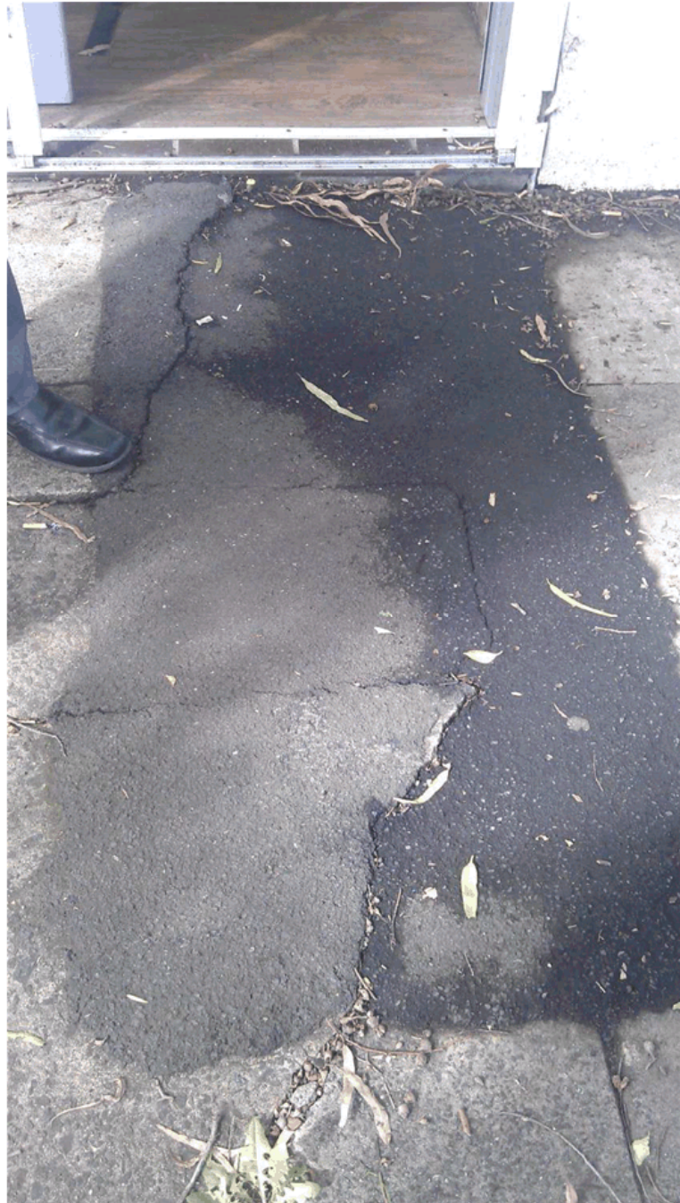
Damage from the tree leading to the front door of the business at no.2 Vincent St. Note the disjointing of the door frame with the masonry wall and also the damage to the footpath that has been previously repaired.
