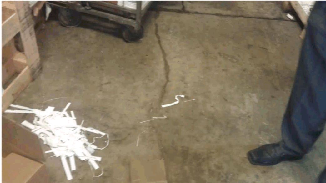
Damage found to the internal concrete areas due to roots penetrating into the property at 2 Vincent St
