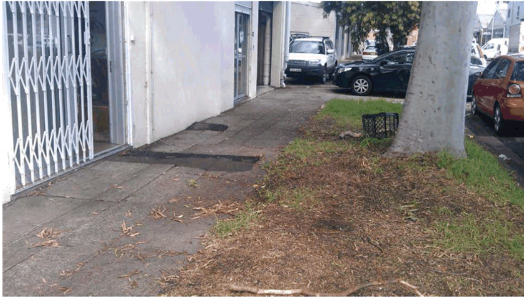
Damage to the footpath leading to the property no.2 Vincent St. Note the Council repairs of the footpath which are now also dangerous trip hazards.
